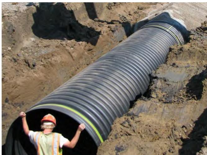
Some corrugated high-density polyethylene (HDPE) pipe is made with a minimum of 40 percent recycled content, taking bottles from curbside collection to lifelong underground infrastructure improvement.
